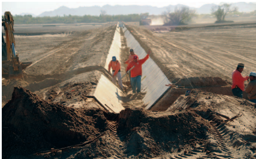
Initial work included clearing and burning of non-native vegetation, excavation of historic channels, and the installation of water control structures. Here, I&R Contracting puts the finishing touches on irrigation ditches and laser-leveled fields, which were then planted with cottonwoods, willows, mesquites, and a variety of other native plants. Freshwater pumped from the river and used for flood irrigation provided the best scenario for establishing native riparian species. Photo by Fred Phillips
