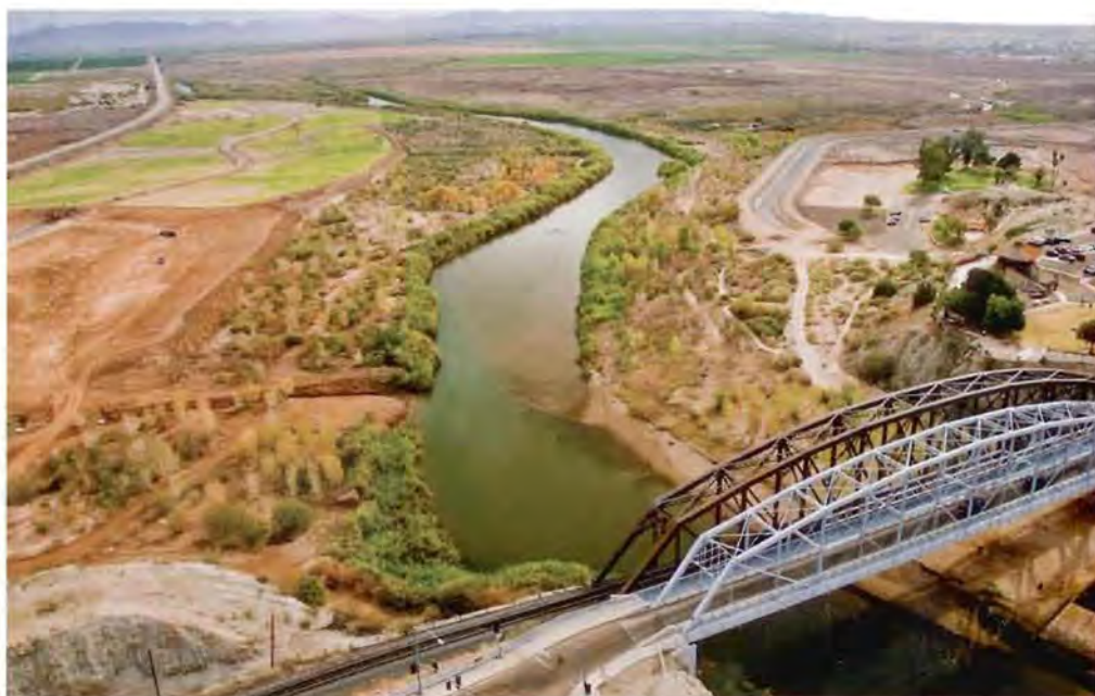
An aerial view from above downtown Yuma at Ocean-to-Ocean Bridge shows agricultural fields just cleared of tamarisk, ready for flood irrigation, on the left, and riverbanks and wetlands three years after restoration on the upper right.
