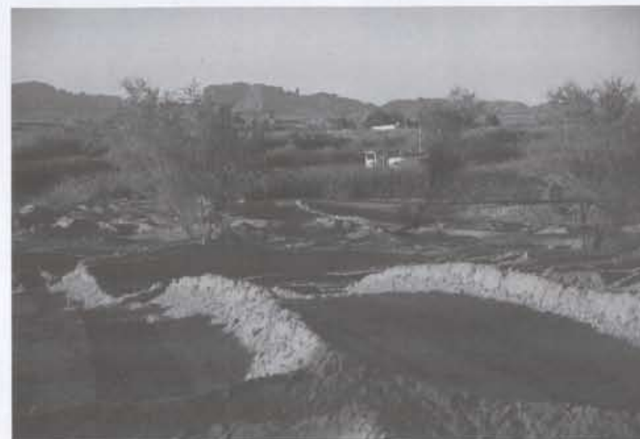
Dredge spoils removed from backwater of Colorado River create windrows on-site at 'Ahakhav Tribal Preserve. Graded to match contours of the site, spoils provide good medium for planting of native species, following pin-point prescription based on high-resolution mapping of hydrology of planting sites. Photos by Fred Phillips
